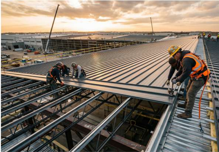
STANDING SEEM ROOF INSTALLATION
