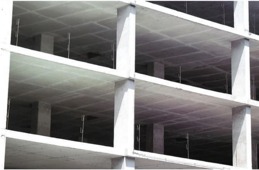
CONVENTIONAL CONCRETE SLAB
